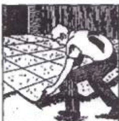
Lay out the tiles dry
